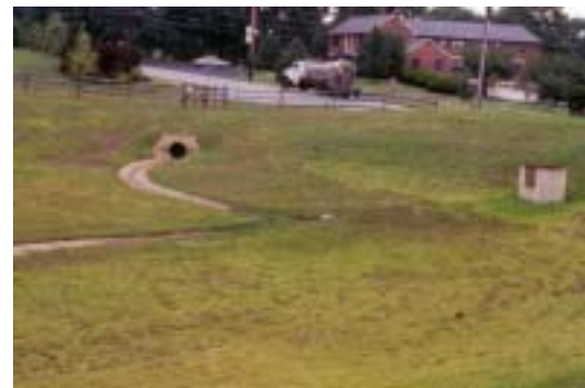
A traditional stormwater detention basin.
